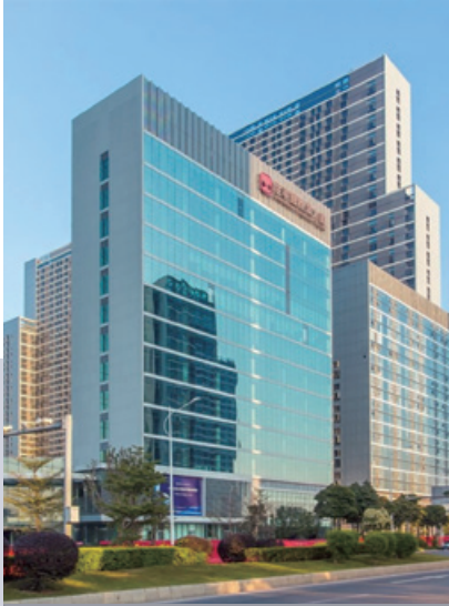
Carrianna Business Centre at Guangzhou South Station 廣州南站佳寧娜商業中心
