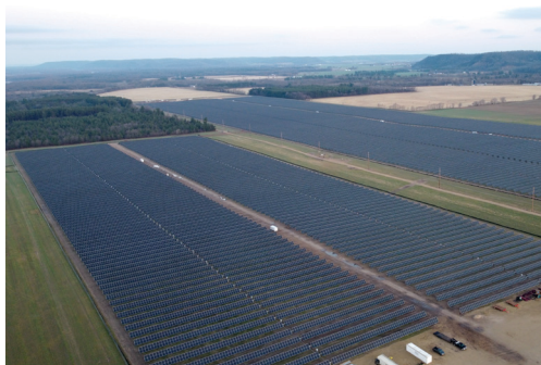
Bear Creek – 50 MW project
