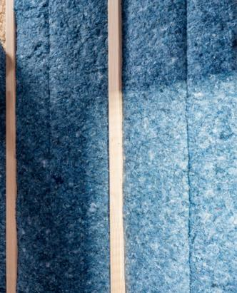
Henry UltraTouch<sup>™</sup> insulation is crafted from 80% recycled denim, lowering environmental impact and streamlining installation time without compromising performance
