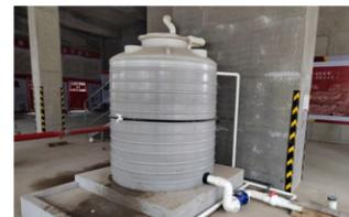
Rainwater collection tanks installed at the site of the Changsha North Star Delta A2 Project, for using the water collected for on-site dust reduction, water spraying, and washing machine water replenishment
