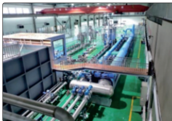
Large-Scale Water Loop Test Facility
