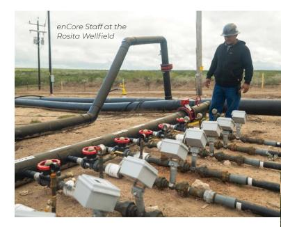
chemistry and hydrology to assure there are no impacts to any adjacent underground sources of drinking water. The combination of the production patterns and the monitor well network constitute what is called a wellfield
