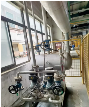
Steam Condensate Water Recovery System
