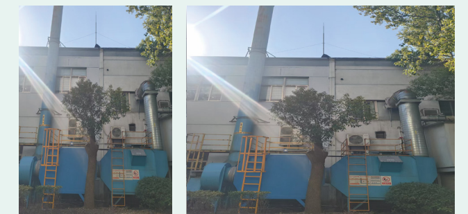
SuperMix Waste Gas Treatment Equipment
