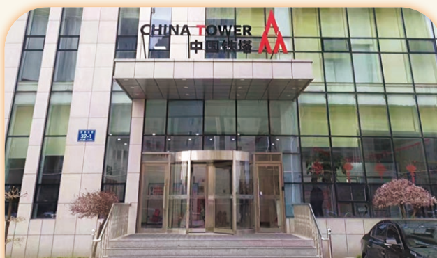
遼寧錦州鐵塔 China Tower Liaoning Jinzhou Branch
