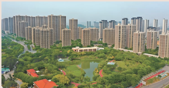
廈門洋唐居住區保障性安居工程項目 Xiamen Yangtang Residential Area Affordable Housing Project
