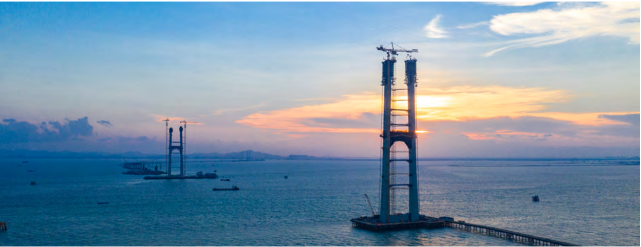
一体化智能筑塔机应用于深中通道伶仃洋大桥 Integrated intelligent tower building machine used at the Shenzhen-Zhongshan Link and Lingdingyang Bridge
