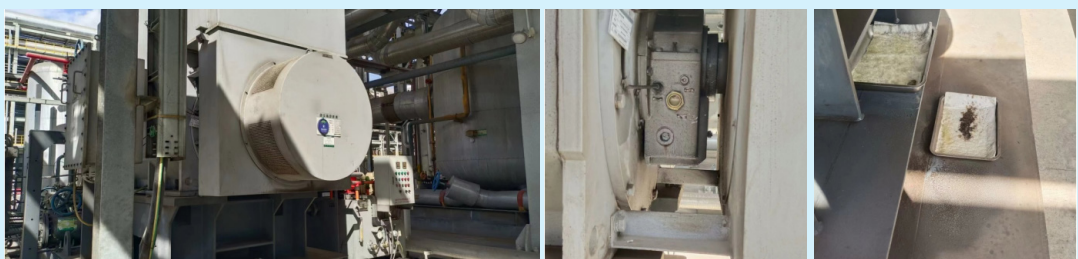
Oil Leakage at the Shaft Penetration Of the Tail Bearing
