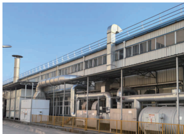
Centralized Welding Fume Collection and Treatment Equipment
