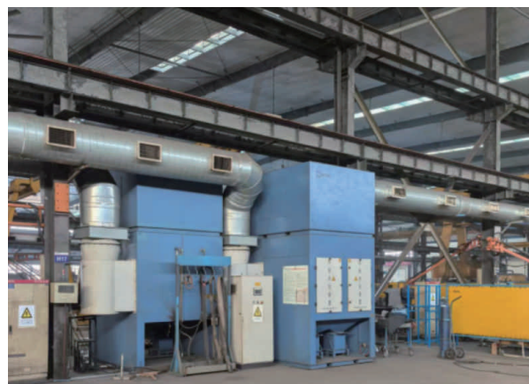
Painting Workshop Equipped with VOCs Collection and Treatment Systems
