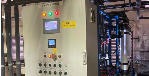
Ceramic Ultra Filtration membrane, recycling of organic wastewater
