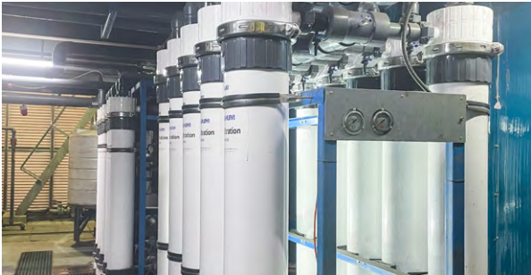
Ultra Filtration membrane, recycling of grinding wastewater
