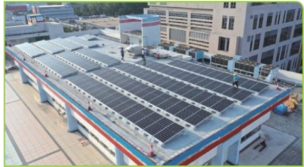
◇ The 220-kW solar PV modules installed at the roof top of Lam Soon Building in Hong Kong 於香港南順大廈的屋頂所安裝220千瓦的太陽能光伏組件
