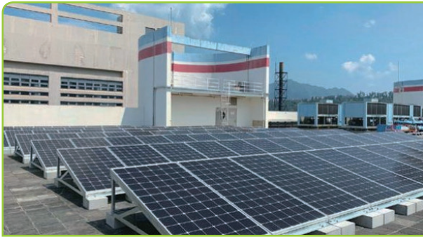
◇ The 220-kW solar PV modules installed at the roof top of Lam Soon Building in Hong Kong 於香港南順大廈的屋頂所安裝220千瓦的太陽能光伏組件
