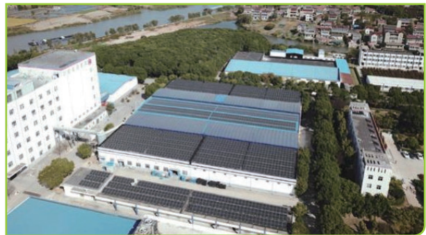
◇ The 220-kW solar PV modules installed at the roof top of Lam Soon Building in Hong Kong 於香港南順大廈的屋頂所安裝220千瓦的太陽能光伏組件
