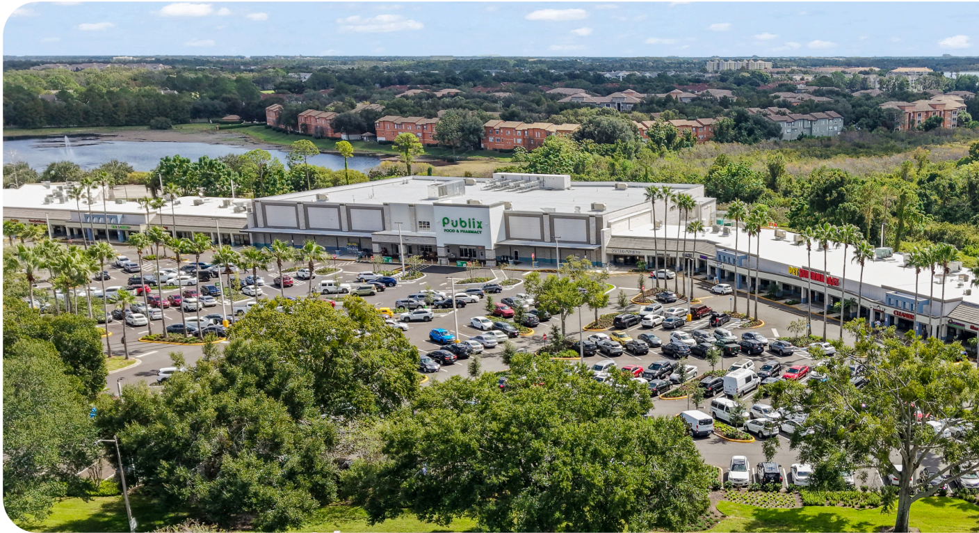
MetroWest Village | Orlando, FL
