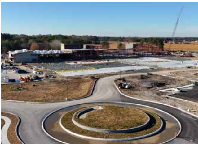
SUSSEX COUNTY VOCATIONAL TECHNICAL SCHOOL CONSTRUCTION
