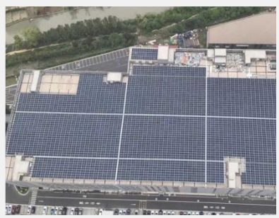
Roof Photovoltaic of Ninebot (Changzhou) Technology Co., Ltd.
