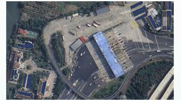
甬台温高速温州服务区光伏布局 Photovoltaic layout of the Wenzhou Service Area, Ningbo-Taizhou-Wenzhou Expressway
