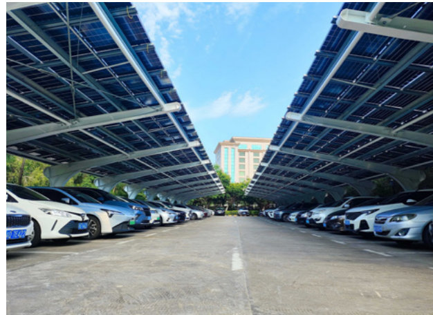
Shantou Port adopts building-integrated photovoltaics (BIPV) to construct a photovoltaic carport
