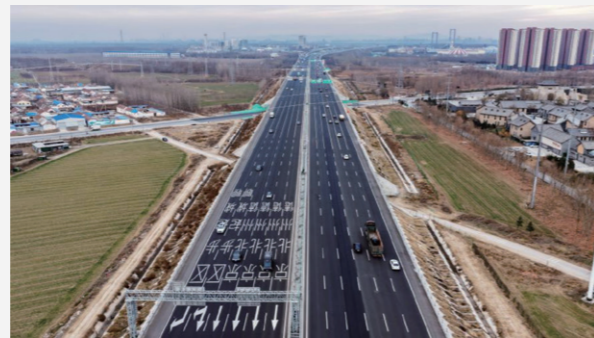
Beijing-Taipei Expressway Reconstruction and Expansion Project
