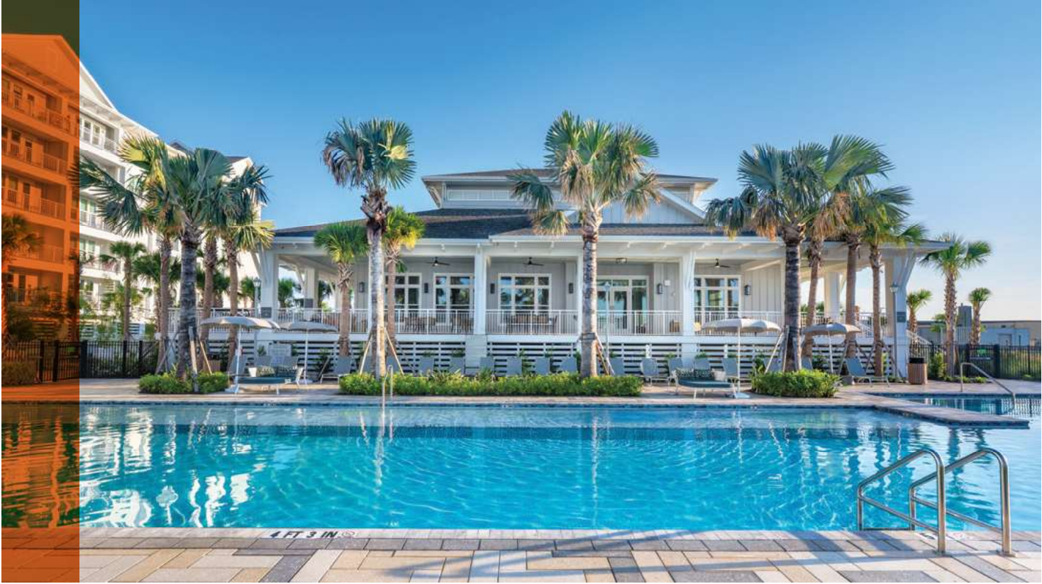
MAA Breakwater, Tampa, FL
