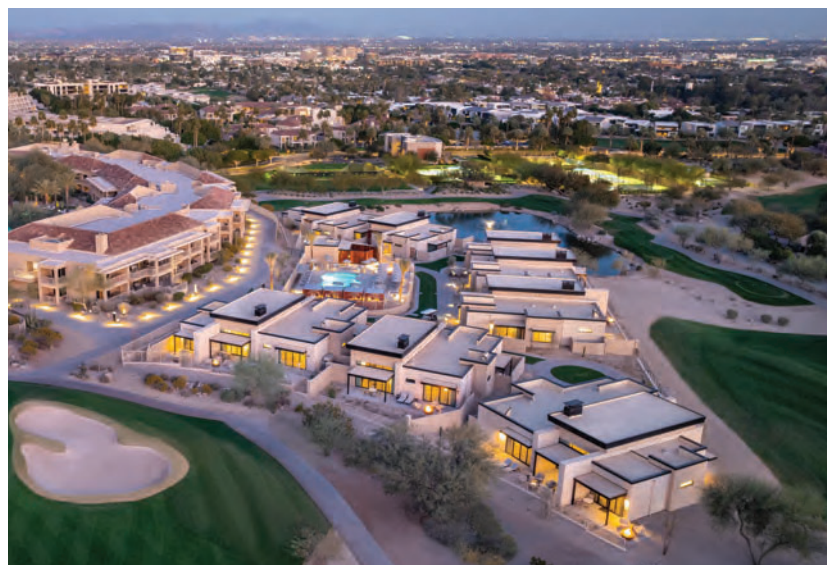
THE PHOENICIAN, A LUXURY COLLECTION RESORT, SCOTTSDALE (20-Key Villas Expansion Completed in January 2026)
