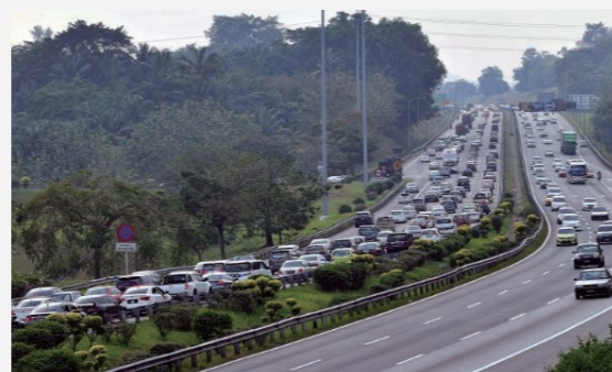
PLUS Expressway Expansion Project
