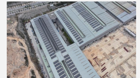
Distributed PV Power Station
