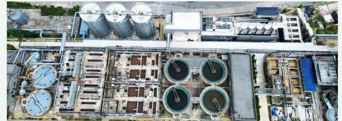
Renovation and Upgrading of the Sewage Treatment Plant
