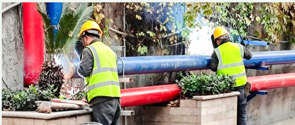
Water-Saving Pipeline Renovation Site
