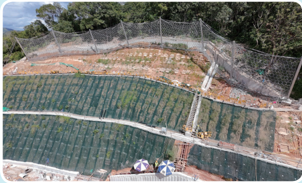
Site Formation Works at Queen's Hill Extension, Fanling
