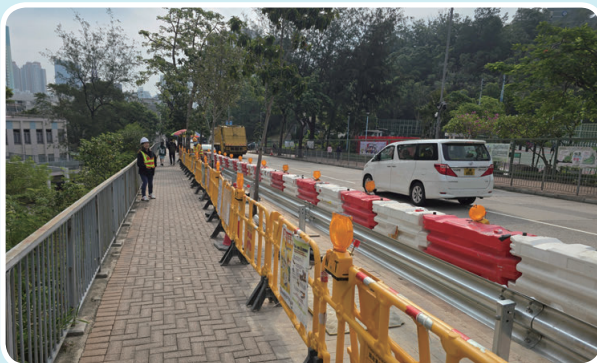
Description: Construction of safety fence beam
