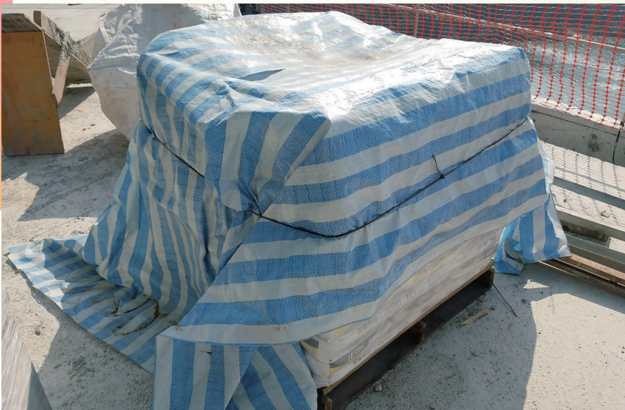
Cover the Stockpile of Dusty Materials 覆蓋易生塵埃的物料堆
