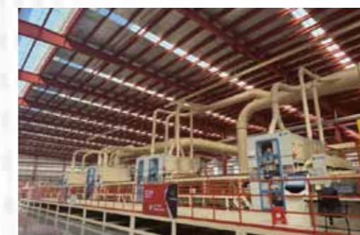
Integrated production line for sanding, sawing, sorting and packaging of wood-based panels
