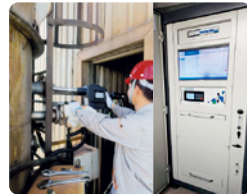
Installation and Networking of Monitoring Equipment
