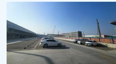
Construction of a New Parking Lot
