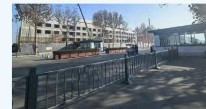
Installation of Pedestrian Guardrails
