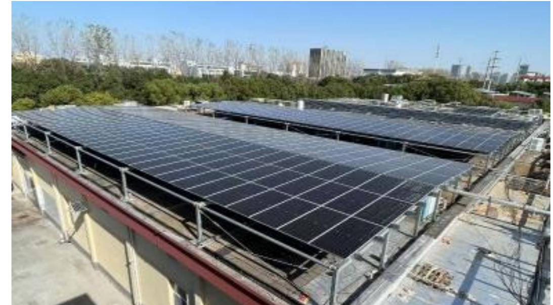
Installing rooftop PV systems
