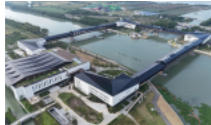
“一点”方厅水院光伏及光储直柔工程
