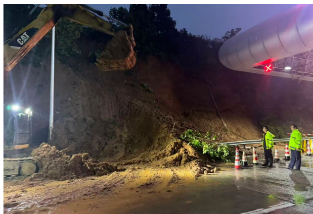
边坡滑塌应急抢险
