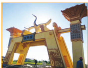
Large Scale Outdoor Structure 大型戶外構築物
