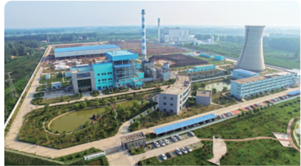
Dangshan Integrated Biomass and Waste-to-Energy Project 碭山生物質及垃圾發電一體化項目
