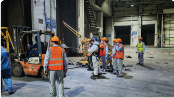
Boluo Waste-to-Energy Project conducted confined space emergency rescue drills 博羅垃圾發電項目開展有限空間應急救援演練
