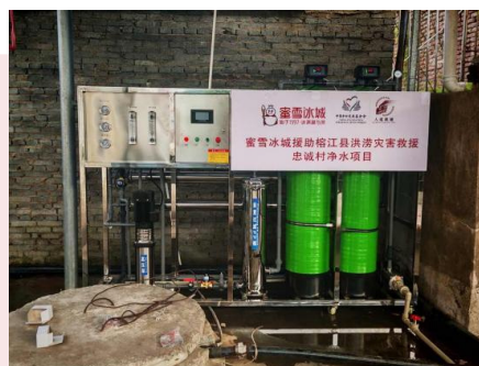
榕江淨水項目 Rongjiang Water Purification Initiative
