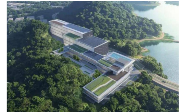
Secondary-side Liquid Cooling System Integration for a National Key AIDC Project in Shenzhen
