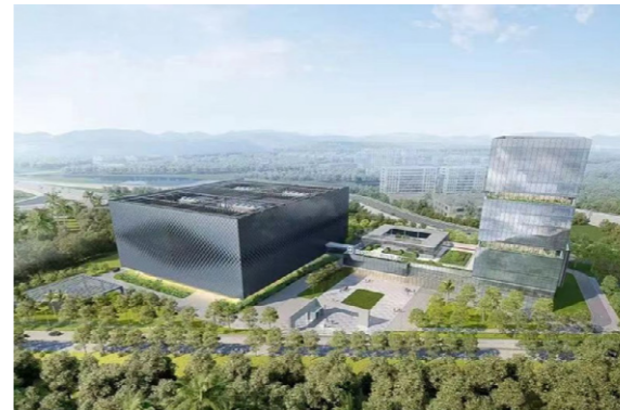
Secondary-side Liquid Cooling System Integration for a National Supercomputing Center
