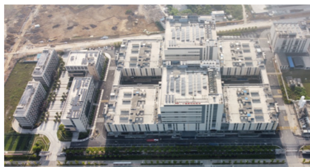
Photovoltaic Rooftop at XWXN (Ningde)
