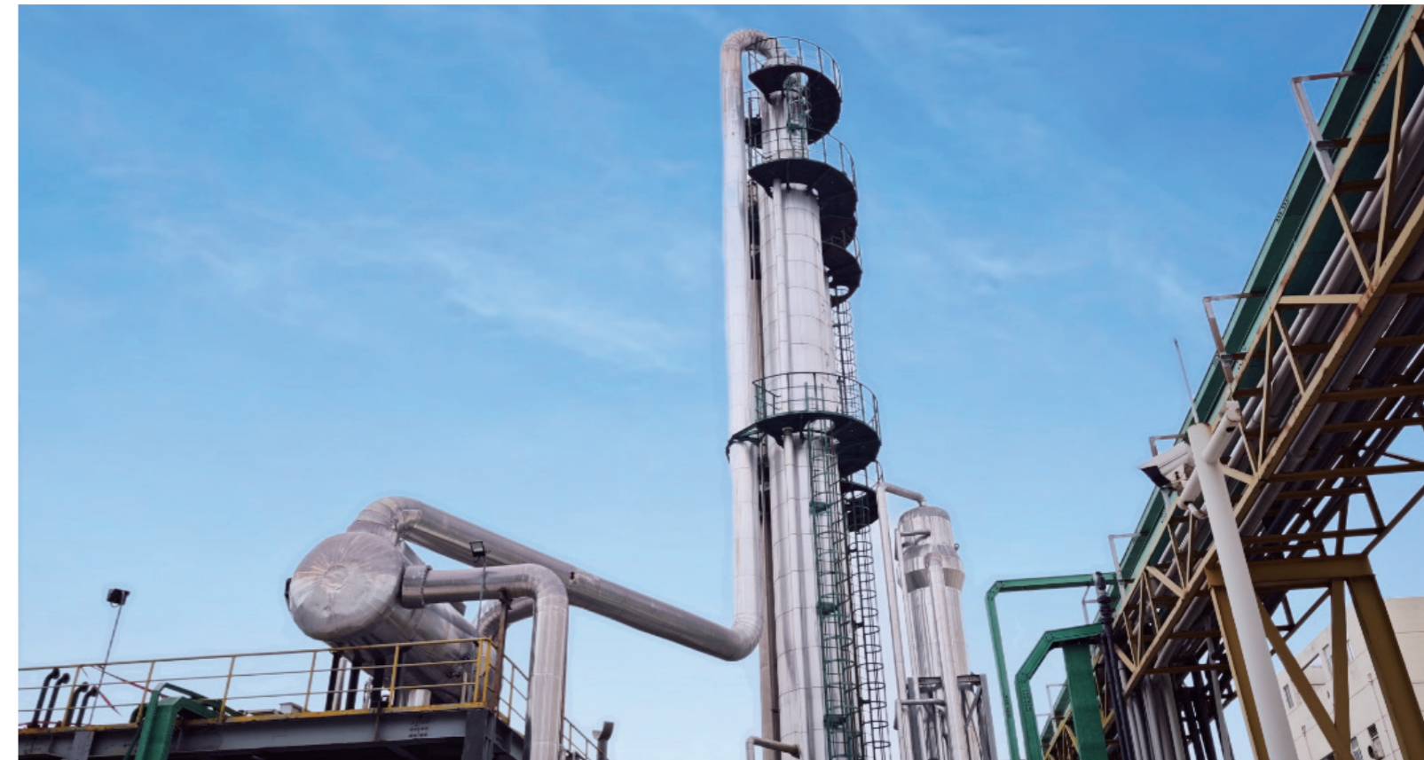
Wastewater Treatment Facilities
