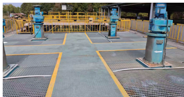
Water Treatment Facilities
