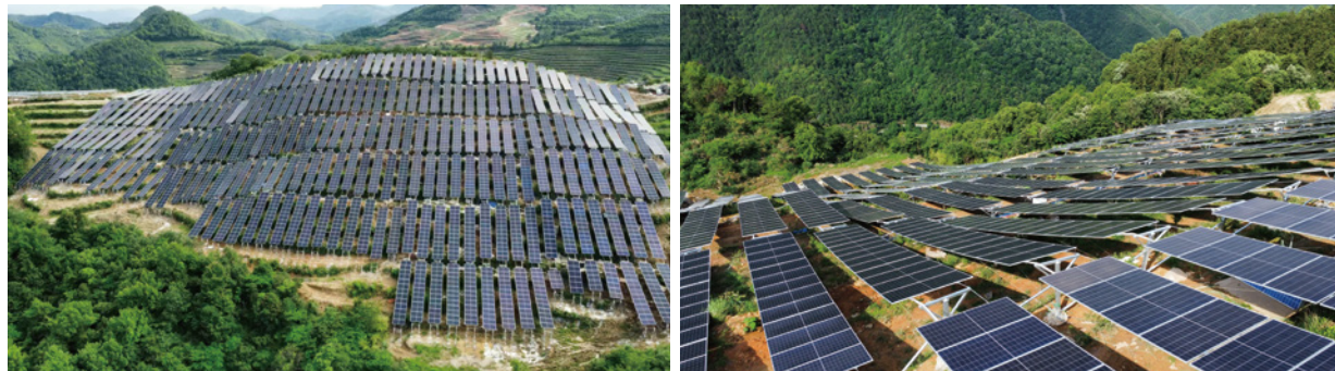
“三门县亭旁镇视头村11.98MWp茶光互补EPC项目”
