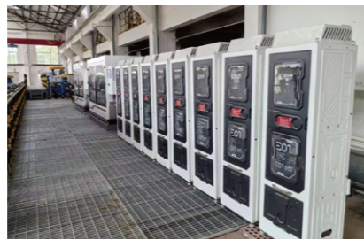
Automated Reagent Dosing System for Flotation
