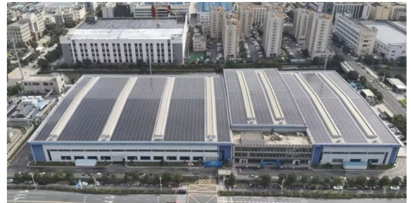
↑ Building Rooftop Photovoltaic Photo
