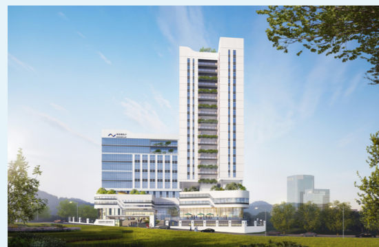
Shenzhen Industrial Base (Under Construction)
