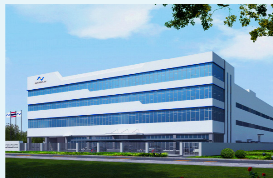
Thailand Production Base (Under Construction)
