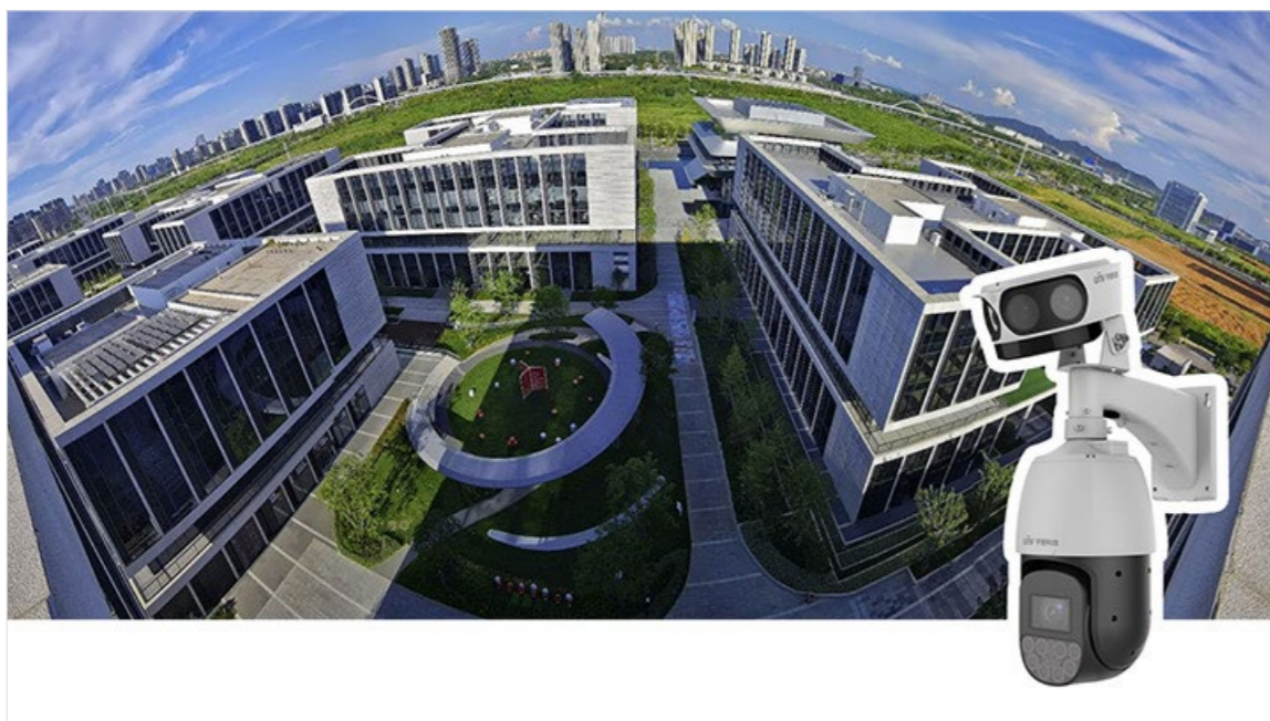
Uniview safeguards Wuhan Jinshan Software Park day and night
