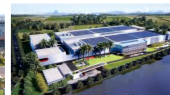
Thailand Kinwong (Under Construction)
