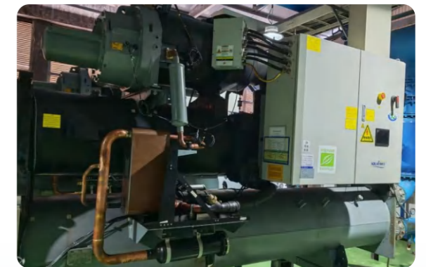
© Central Chiller Station High-Efficiency Plant Room Comprehensive Modification Project
