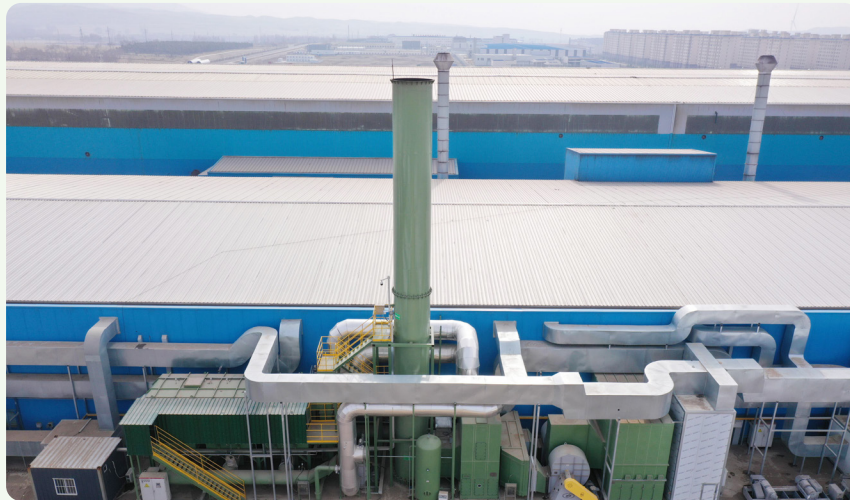
Upgrading of VOCs Treatment Equipment at Zhangjiakou Facility
