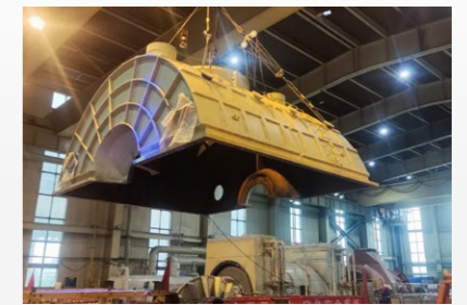
2x300MW low-carbon and energy-efficient comprehensive utilization upgrade project
