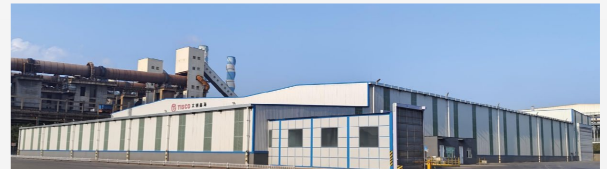
Expansion and enclosure project of the alloy material warehouse at Shandong Taigang Xinhai Stainless Steel Co., Ltd.'s steelmaking plant
