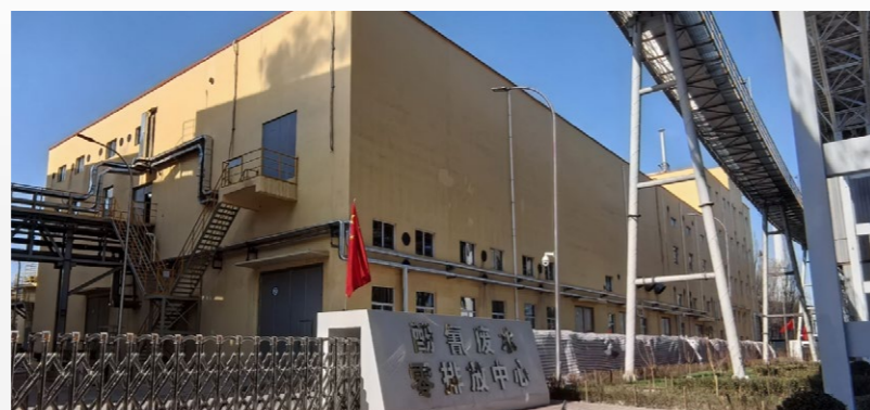
Zero-Discharge Project of Coking Phenol-Cyanide Wastewater
