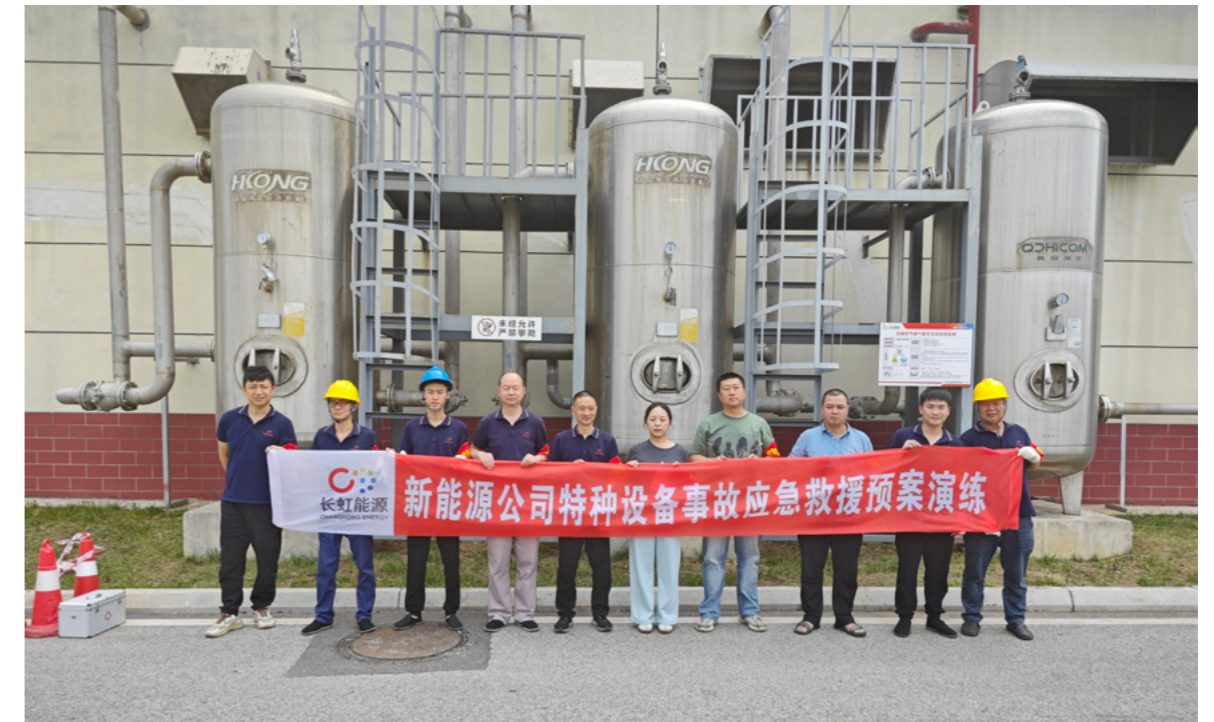
Changhong Newenergy conducts a special emergency drill for special equipment (compressed air tank)
