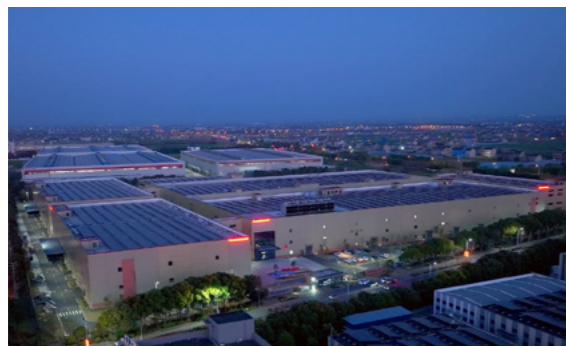
Changhong Sanjie Phase IV Project Production Workshop
