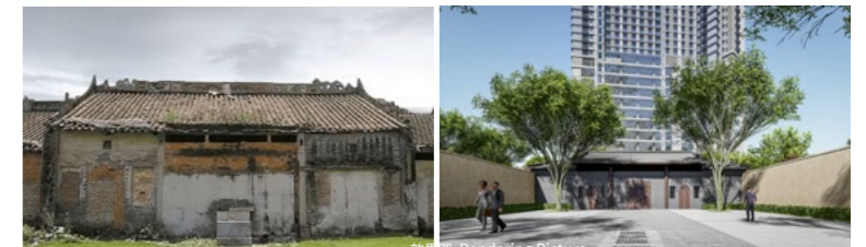
深圳遠洋濱海大廈春牛堂修繕前後對比 Comparison before and after the renovation of Spring Cattle Hall of Ocean Seafont Towers (Shenzhen)
