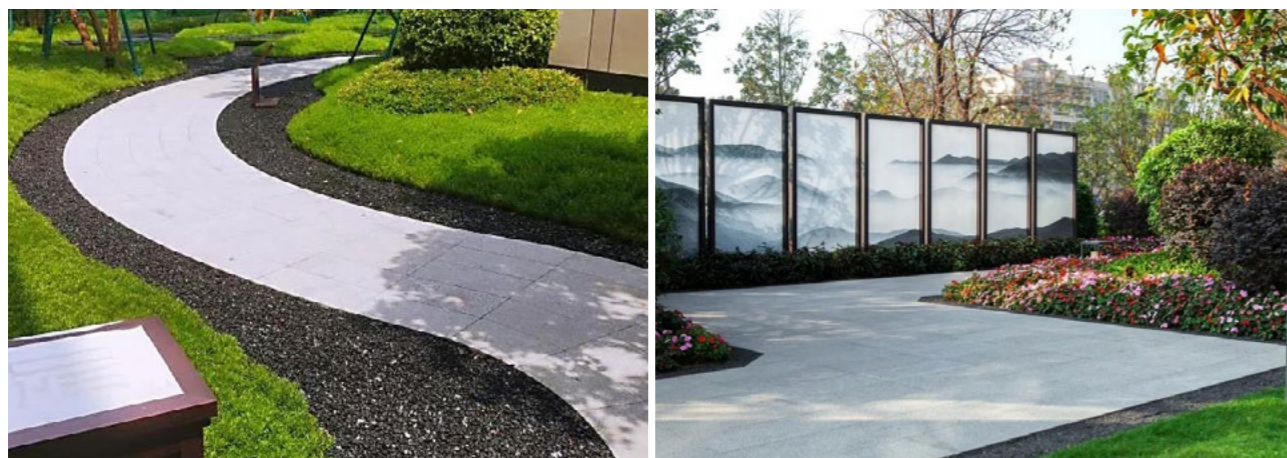
陶瓷仿石磚路面 Pavement surface with ceramic imitation stone bricks
