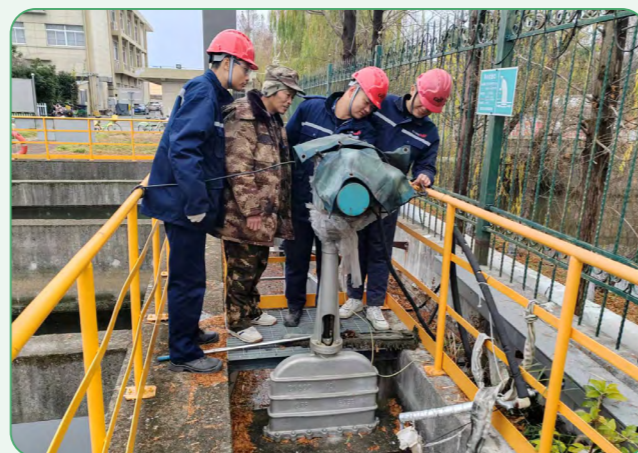
Training Session: Closing a Valve, Plugging a Leak Point
