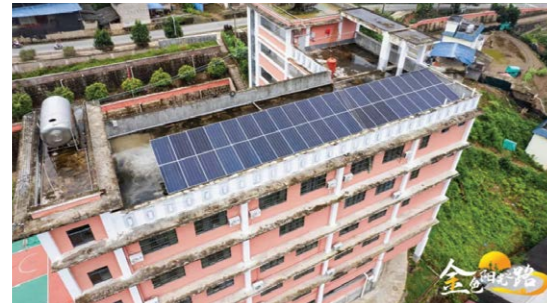
Charity Power Station Project
