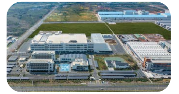
Guangde Factory (Phase I & II, Phase III), China
