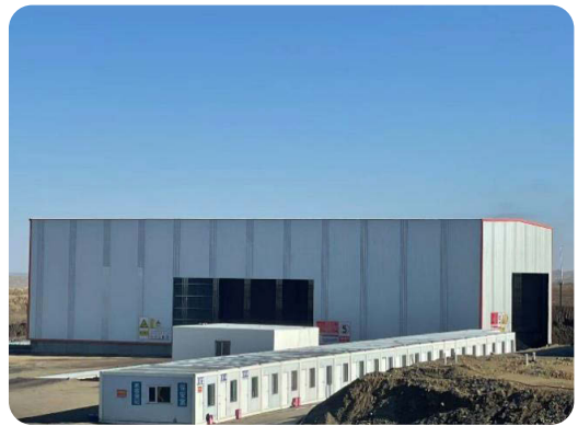
滿都拉口岸新建封閉式煤棚
